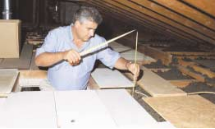
Inspecting the insulation is part of CI's checklist.
